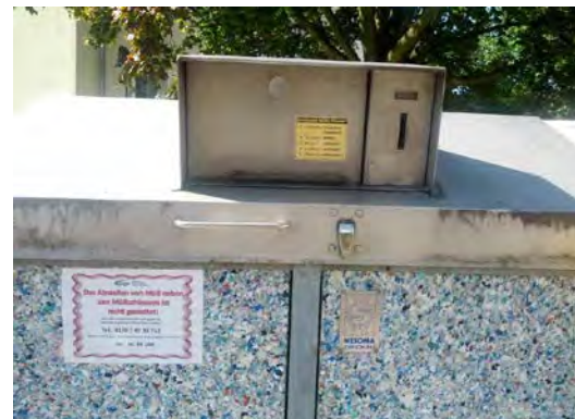
Figure 7: Example for a waste lock with identification system at Wohnungsgenossenschaft „Elbtal“ Heidenau, Germany (photo: S. Guerrero Mercado)
